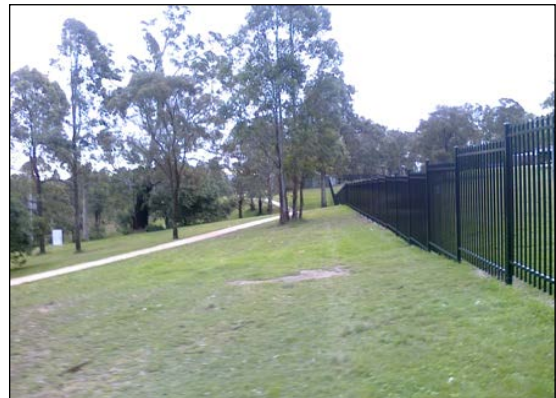
10. View looking west along security fencing
